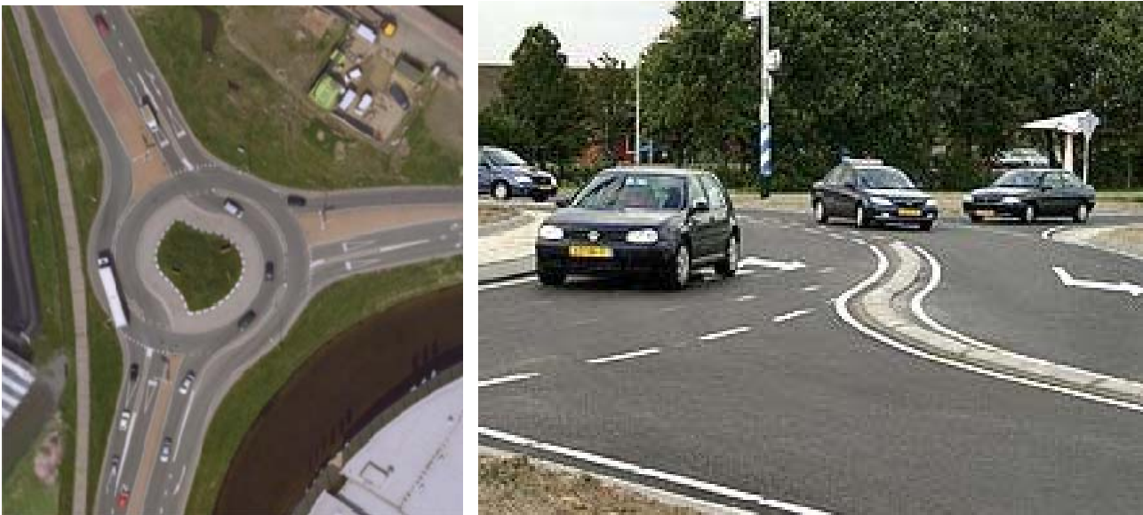
Figure 2: Turbo roundabouts in The Netherlands
