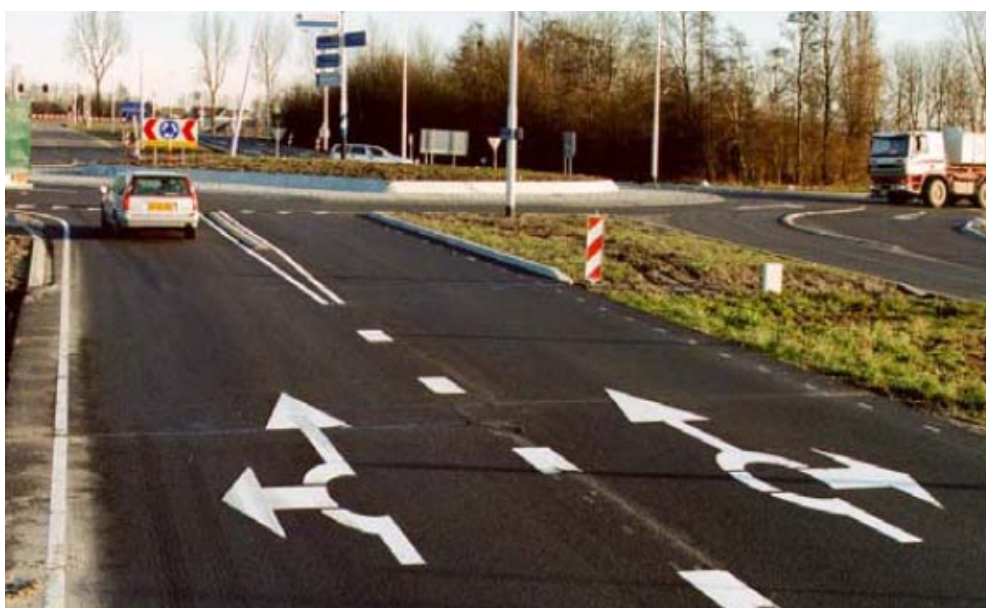
Figure 8: Arrow lane markings especially developed for roundabouts
